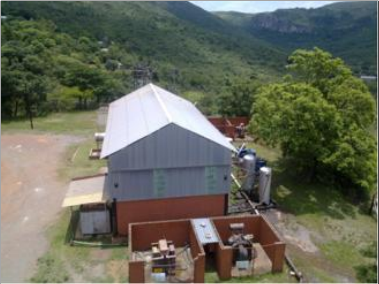
The Compressor Room with Substations and Switchgear
