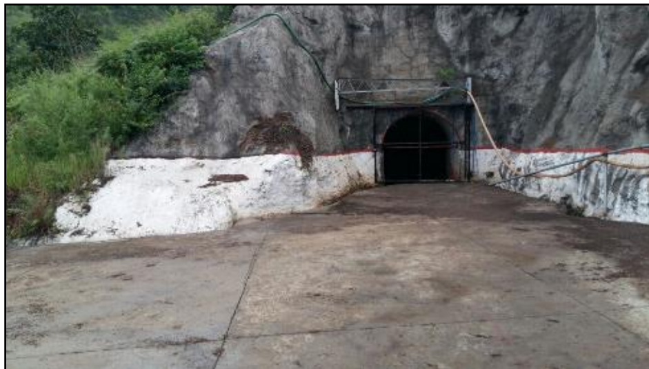
Figure 2) Location of Adit 3 at Rietfontein, refurbished in 2014/15
