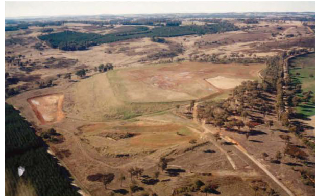
Aerial view of Lucky Draw tailings dam Oblique Aerial Photographs (R.W. Corkery & Co)
